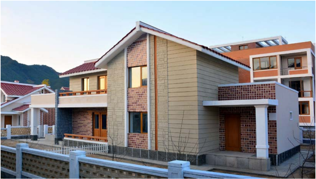
Some of the new dwelling houses in the Mundong Fruit Farm, Pukchong County
